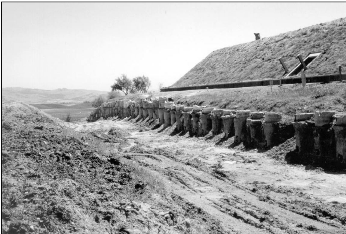
Figure 10. A portion of a tied-back, reinforced concrete shear pin wall installed at the Napa winery site to protect the upslope winery facilities. This shear pin wall roughly follows the alignment of cross-section 1 shown in Figure 7.
